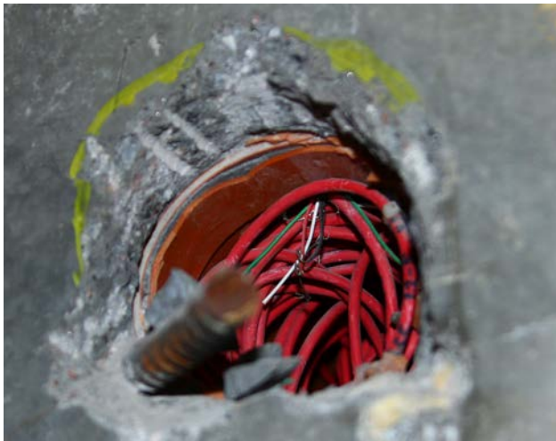
Fig. 11: Embedded detail in BF diaphragm wall after formwork removal
