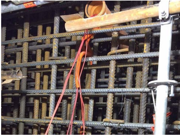
Fig. 8: Embedded PVC details for gauge signal cables
