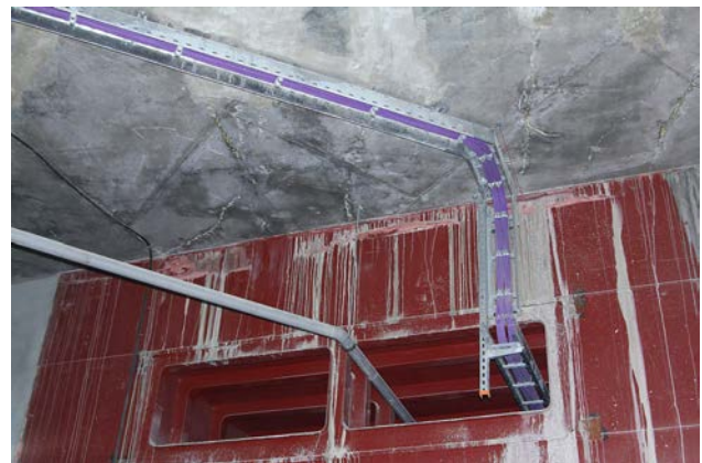
Fig. 17: The supporting system of gauge cables
