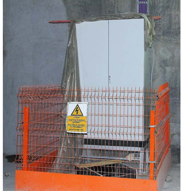
Fig. 12: BF data acquisition enclosure
